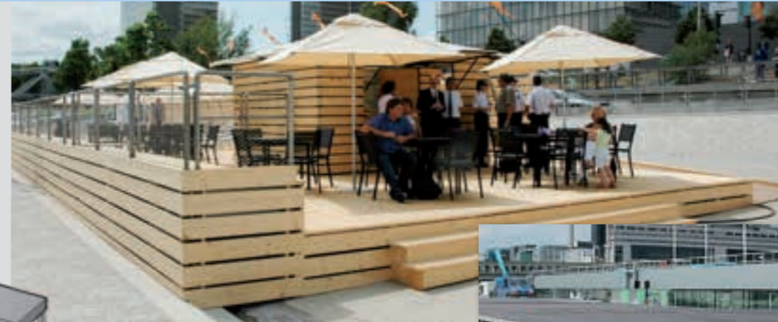
Tanning salon on the Seine in Paris A fourfold underlay, with adjustable elevation, is used as a sub-structure for our Praktikus1000 stage element. The floor covering consists of silk screen slabs.
